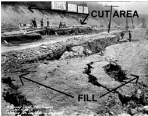
Columbia Avenue in 1930 will soon become Columbia Parkway after it is widened. Photo illustrates early "cut and fill" method of construction in association with a large landslide.
